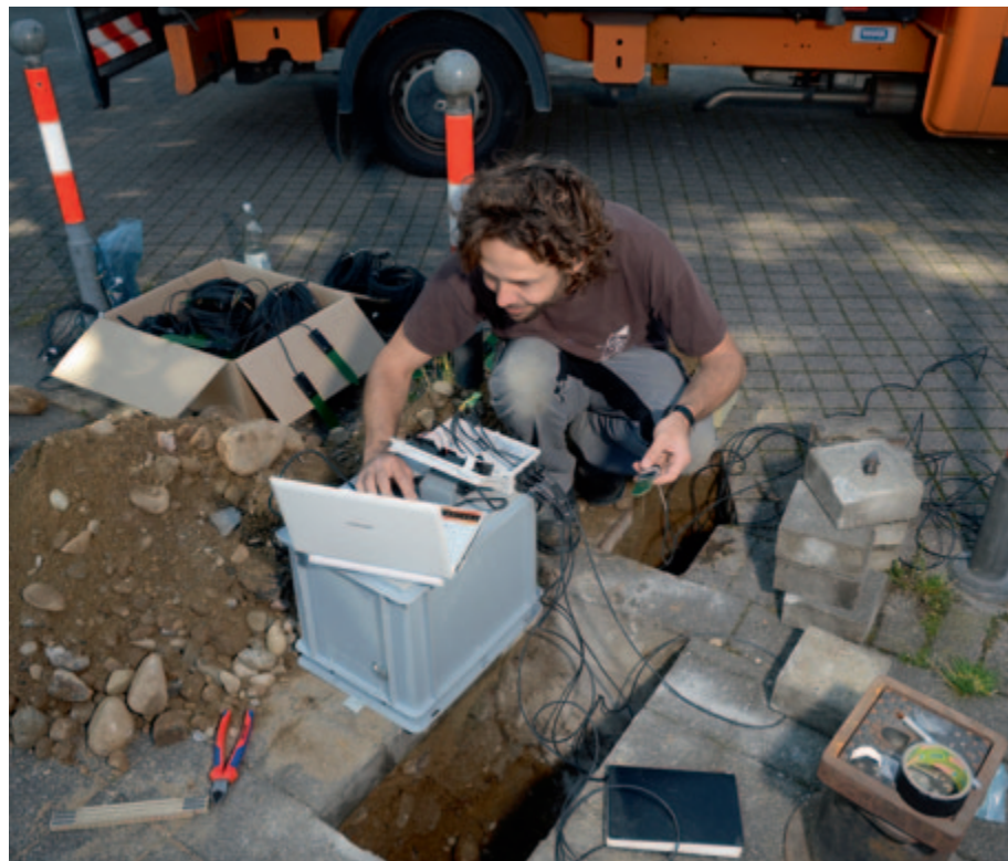
Installation of probes under a paved surface: The hydrologists use the measurement instruments to determine how much it rains and how much of it seeps into the ground or drains off.
